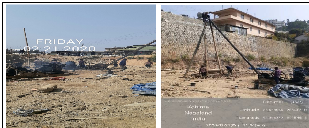
Photograph 6.2: showing the current status of project- TCCC, DH Kohima.
